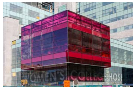
Phase II construction
