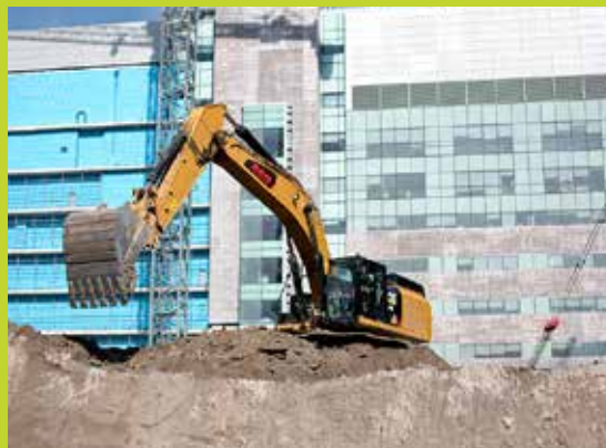
Phase 2 construction under way
